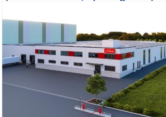
New converting center (Duderstadt site; opening 2020)
