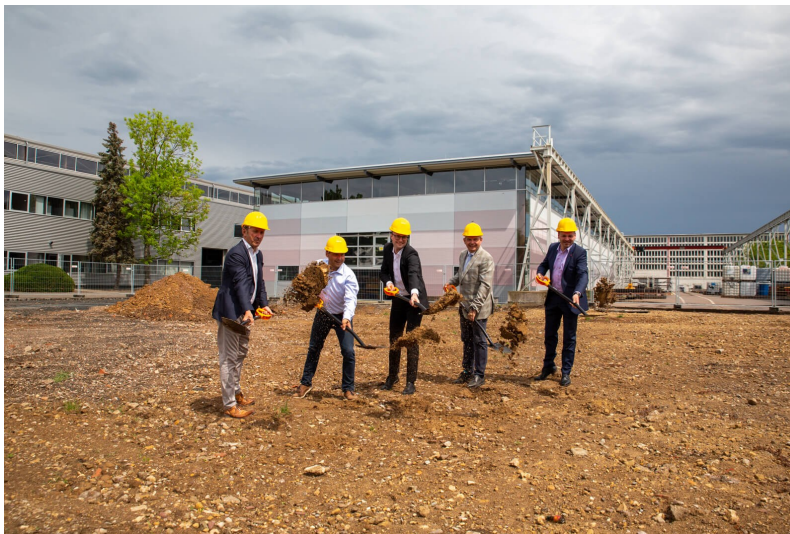
Groundbreaking ceremony for the new ramp-up hall in Gotha with Frank Nosek (Head of Development, Germany), Christoph Rüttimann (CTO), and Daniel Burek (Managing Director, Bystronic Maschinenbau GmbH).
